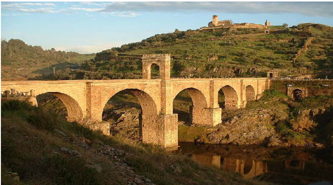
Figure 1.2: Alcantara bridge (2nd century) on Tajo river, mixed masonry, 194m long, 6 spans
