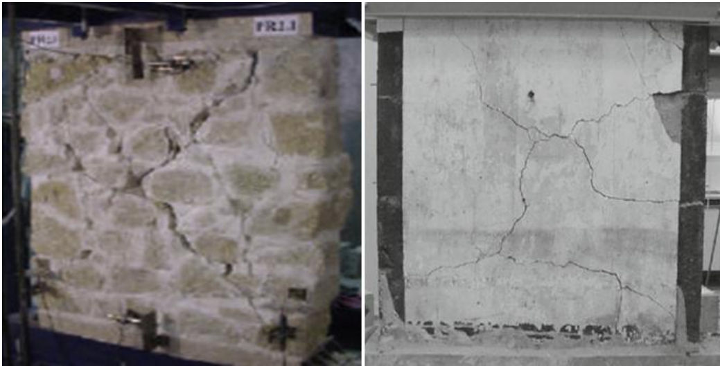
Figure 4.20 Cracking pattern in Actual specimen
