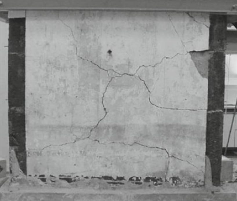
Figure 4.12. Cracking Pattern in actual specimen
