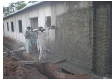
Figure 4.29: Shotcreting and Plaster
