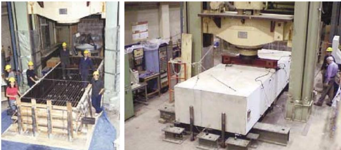
Figure 2.7: Construction and loading of Bahen Centre large wide beam AT-1 under testing machine at the University of Toronto (Lubell et al. 2004).
