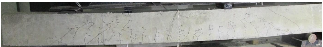
Figure B-20 : Cracking Pattern of C-UR-2
