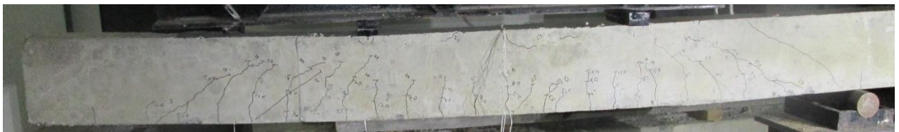
Figure B-27 : Cracking Pattern of C-UR-3
