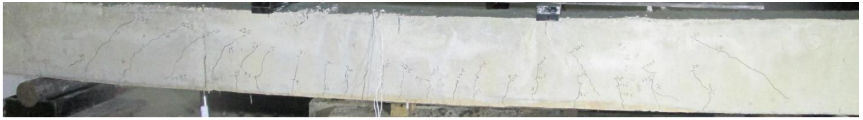
Figure B-19 : Cracking Pattern of C-UR-1
