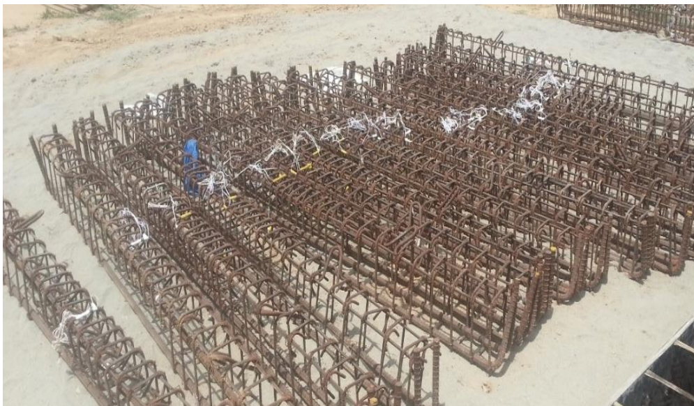
Figure B-5 : Reinforcement Cages For Beams
