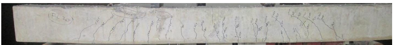
Figure B-23 : Cracking pattern of R-UR-1
