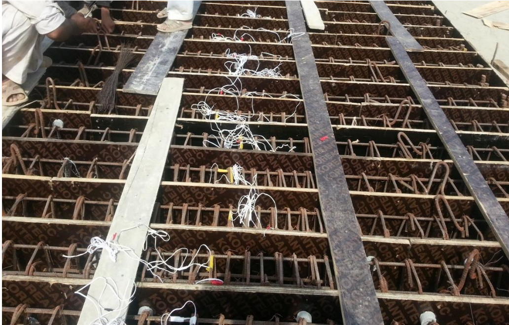
Figure B-6 : Form work for Beams
