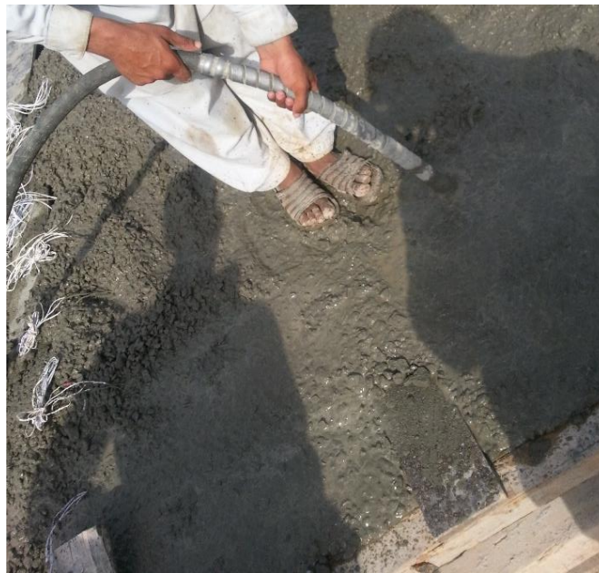
Figure B-7 : Pouring/Casting of Beams
