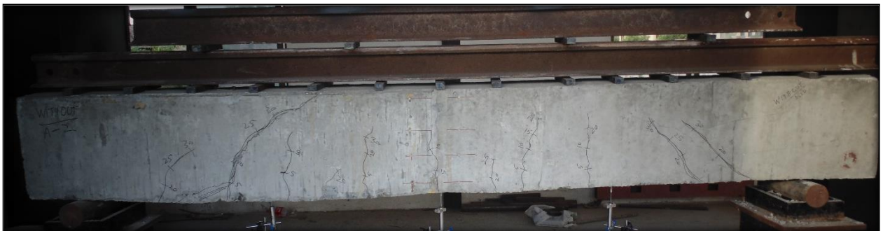
Figure 4-8: Cracked Pattern of N-II
