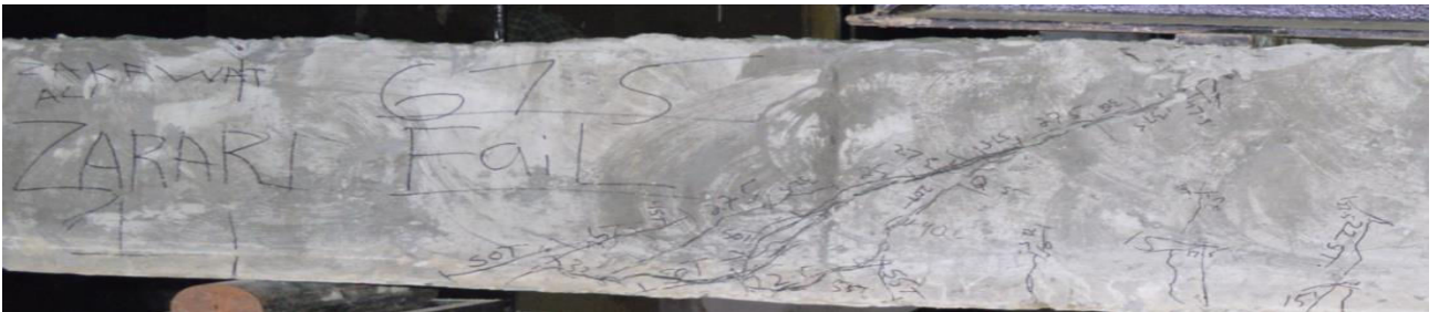
d) West Face South Support
