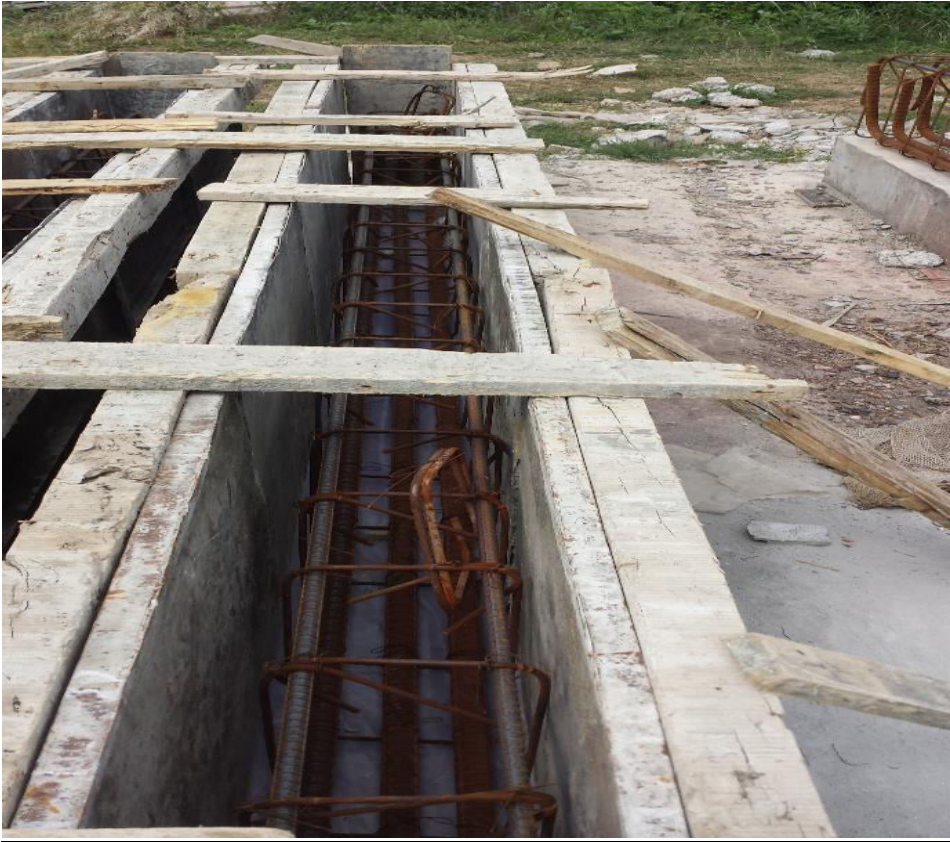
Figure 7: Beam Form work
