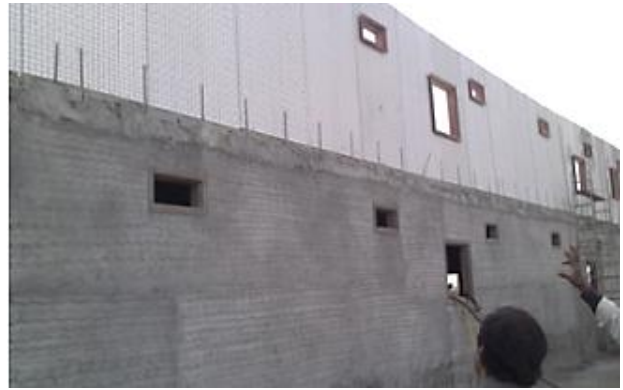
(b). Installation of SCIP panels in the model
