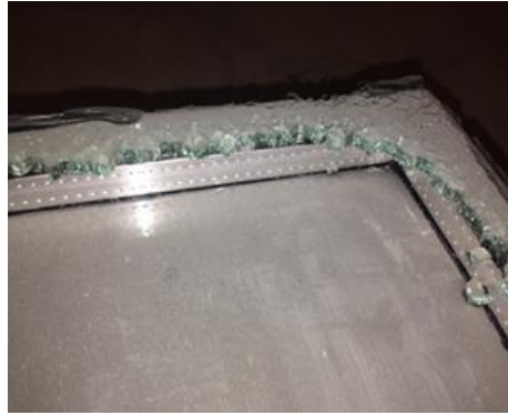
(b) Two layered thick glass with air cavity used in Telecom tower for heat insulation
