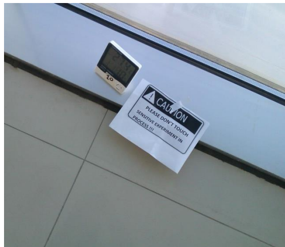
Fig.3.3. Thermometer installed near double layered glass inside Telecom tower
