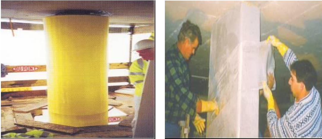
Figure 2-8 Kevlar wrapping (left) and glass wrapping (right)
