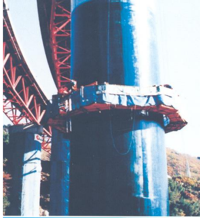
Figure 2-9 Automatic FRP wrapping by means of robot
