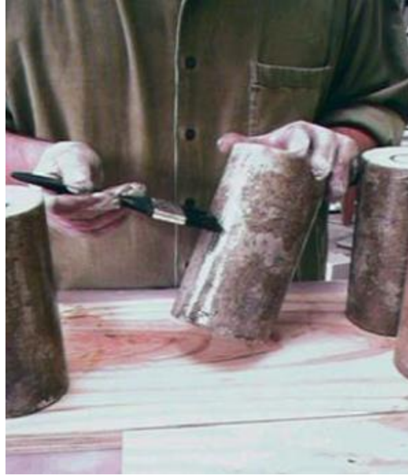
Figure 3-4 Primer epoxy on concrete
