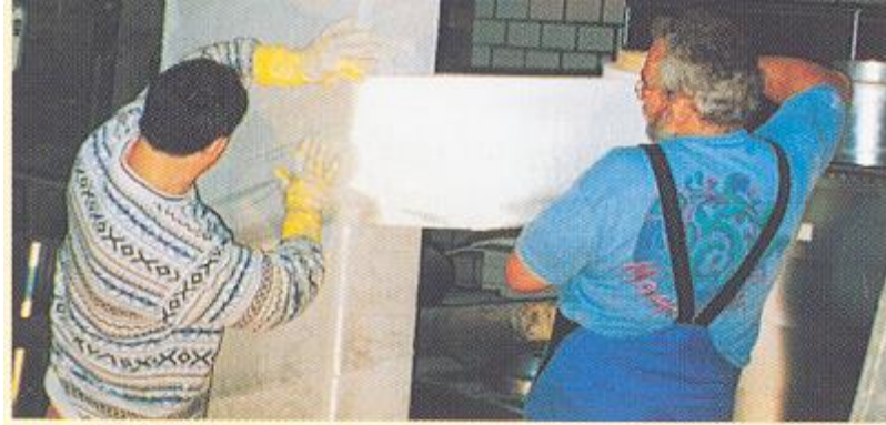
Figure 1-2 Column Strengthening with Glass FRP
