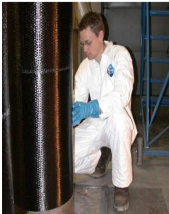
Figure 1-1 Column strengthening with Carbon FRP (left) and Aramid FRP (right)
