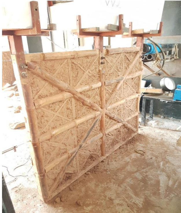
Fig 3.9: DDW2 (Wall Strengthened With Bamboos)
