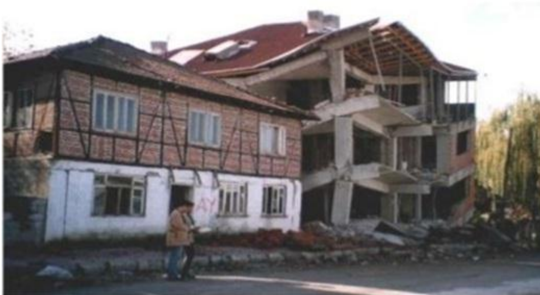
Fig 2.11: An Example of (1999) Turkey Earthquake [12]
