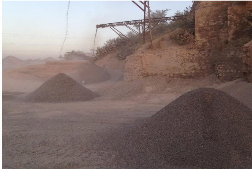
Fig. 3.3 A view of crushing plant from coarse aggregate was arranged (Source: Maragalla)
