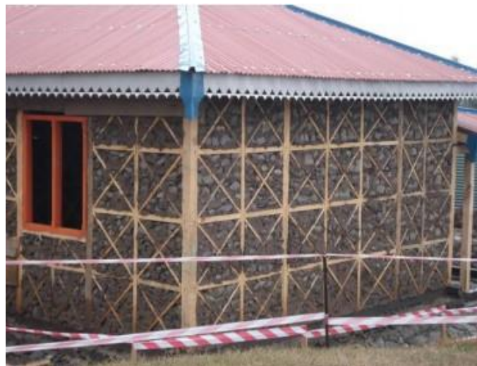
Figure 1.1 Typical Dhajji Dewari House
