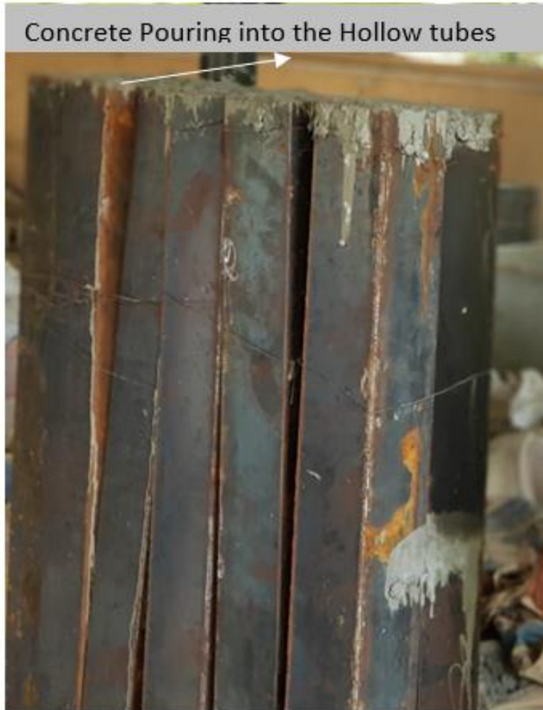
Figure 12: Casting of beams
