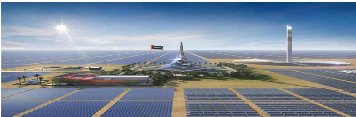
Figure 2.14 Mohammed bin Rashid al-Maktoum Solar Park Phase IV [35]
