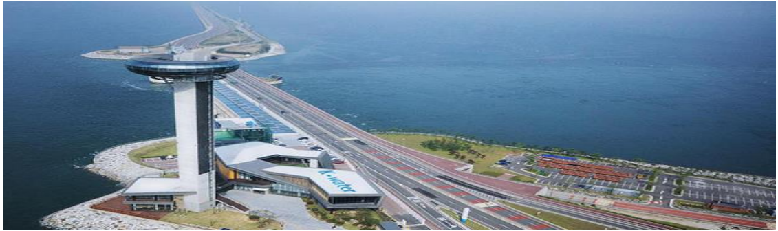
Figure 2.18 Sihwa Lake Tidal Power Station - South Korea [37]
