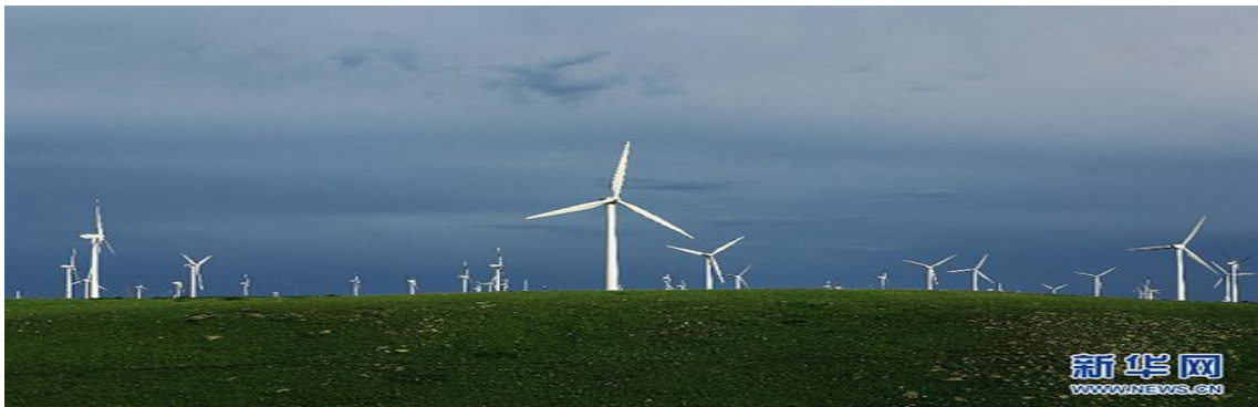
Figure 2.12 Ulanqab Wind Farm [35]
