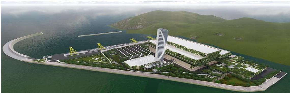
Figure 2.15 Shek Kwu Chau Energy from Waste [35]
