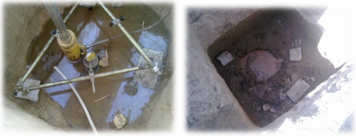
Figure 3.7 Plate load test.
