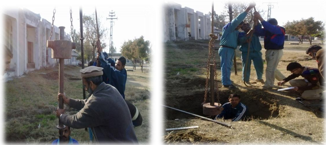
Figure 3.8 conduct of SPT test in test pit# 1.
