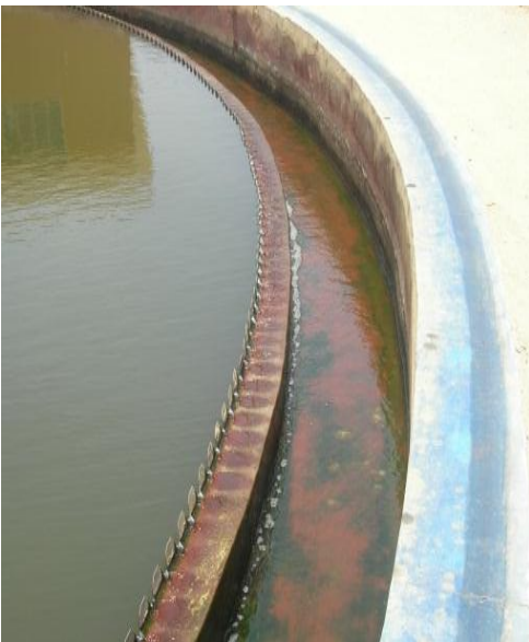
Figure 0-7: Primary sedimentation tank
