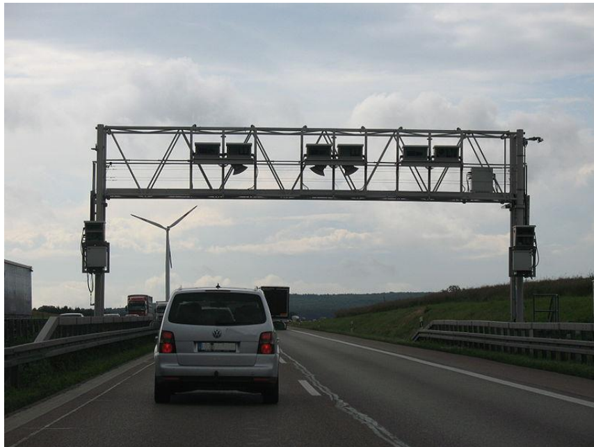
Figure 2-2: A Toll-Collect Gantry on LKW-Maut
