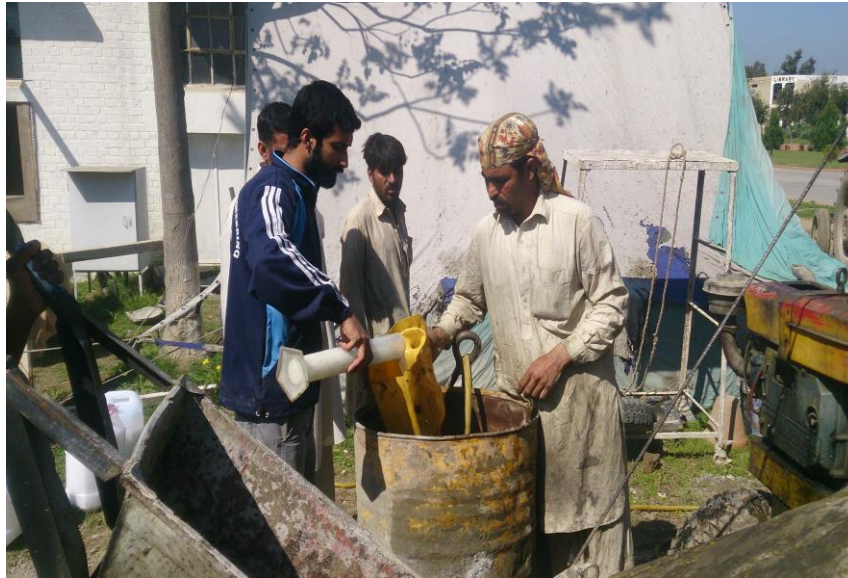
Figure 6.6: Addition of Sika-1 in Concrete Mix during Casting
