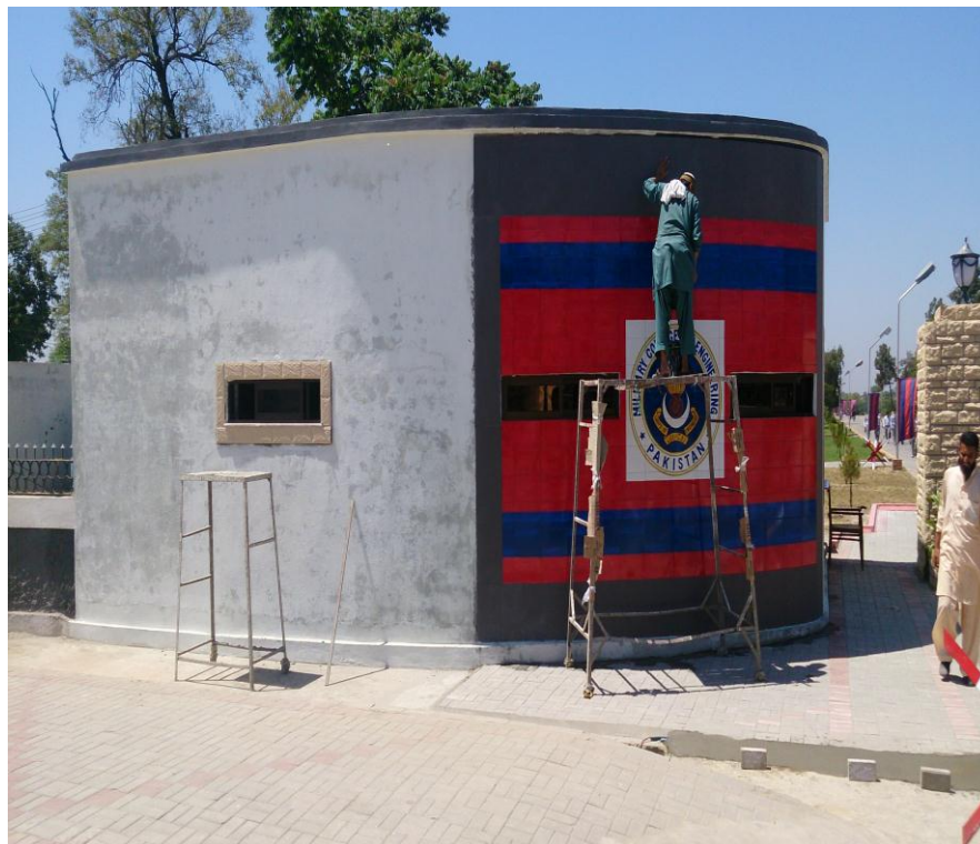
Figure 6.5: MCE gate Guard Room
