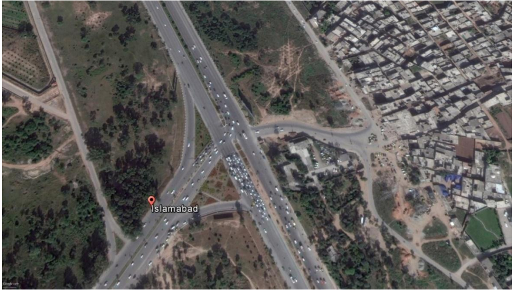
Figure 3.3 Aerial View of Koral Chowk
