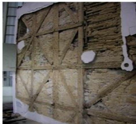
Figure2.9: Gaiola Wall after Test [31]
