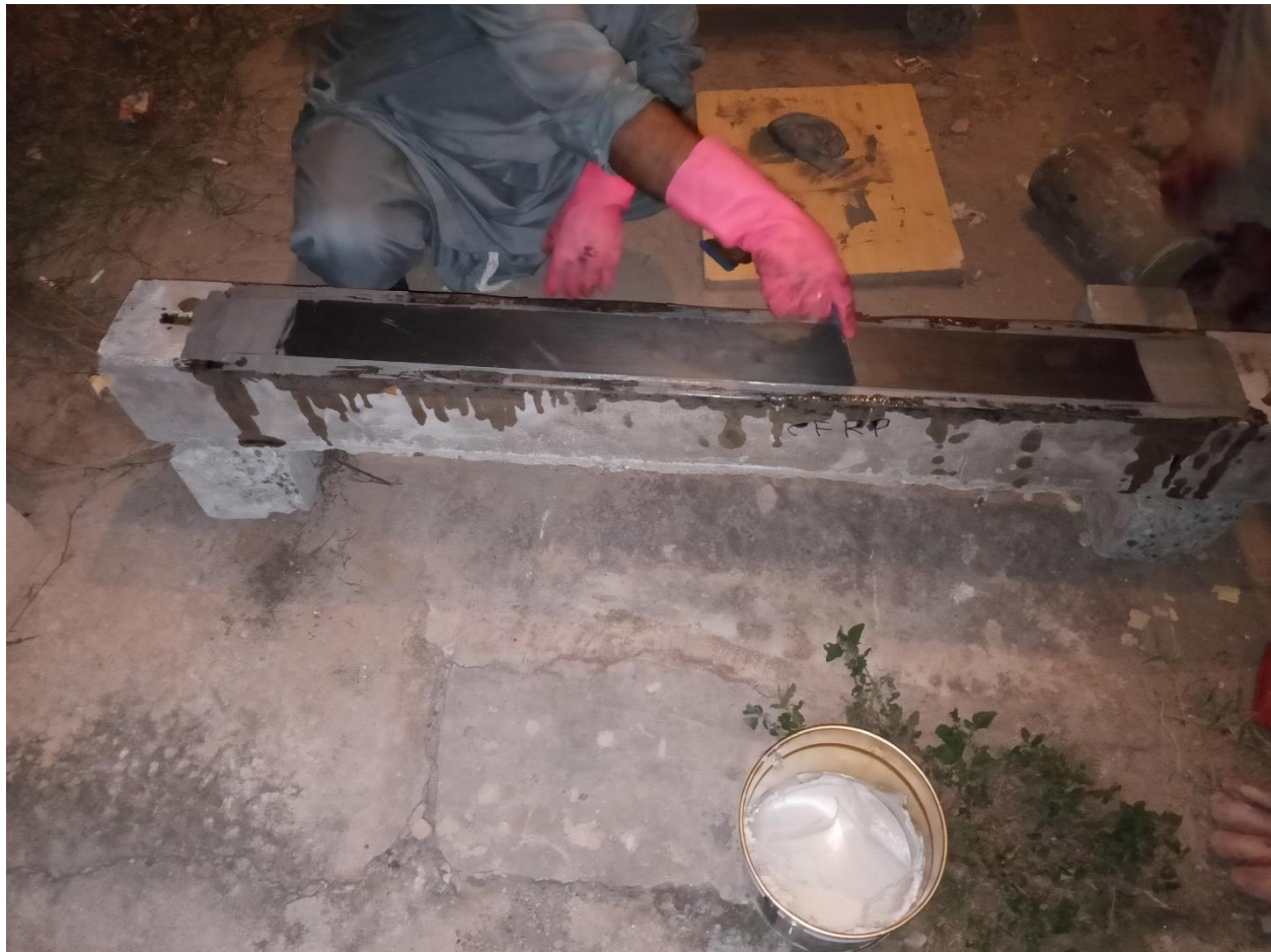
Figure 4.5: Application of CFRP strip
