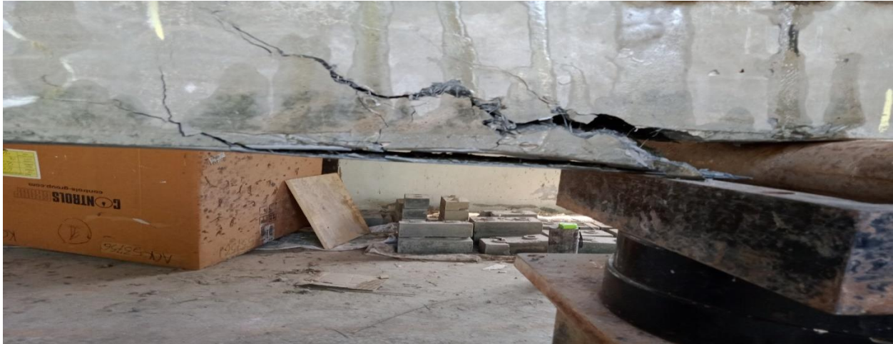
Figure 4.16: Failure pattern of beam with flexural and steel fibers reinforcement along with CFRP (SF-R-C)
