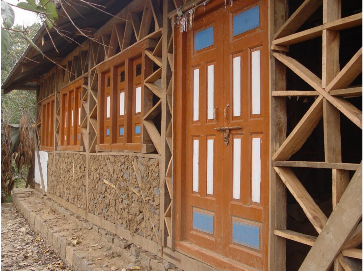
Figure2.1: A Typical Dhajji Dewari House [2]
