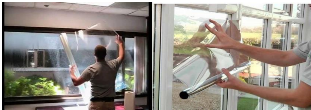
Figure 1.5 Low Emissivity film installation[46]
