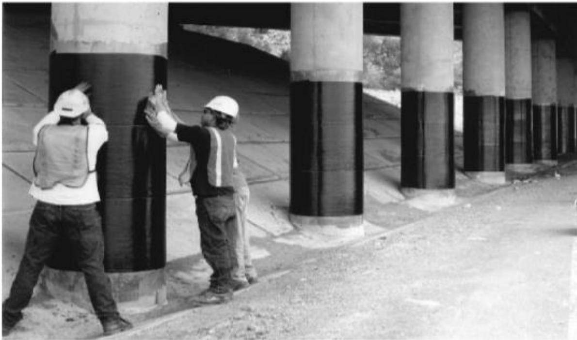
Figure 8: Application of Fibre Reinforced Polymer wrap
