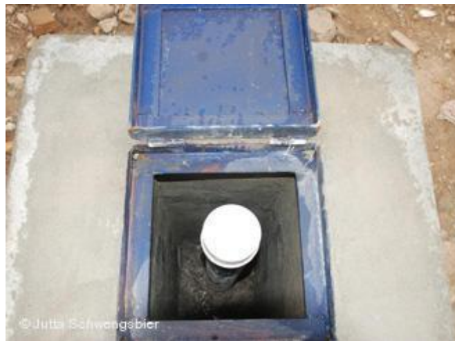
Fig 5.5 Drainage pipes laid to collect water
