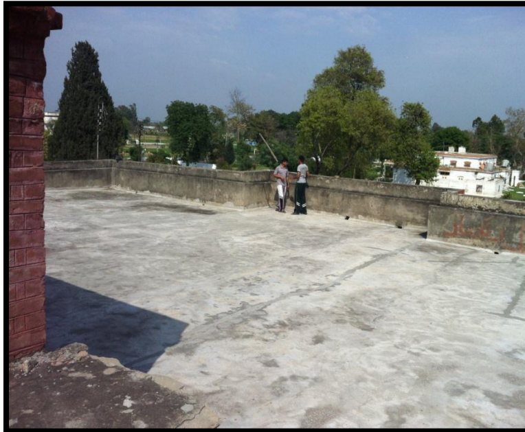
Fig 7.2 Center officers Mess Roof
