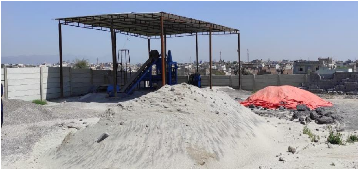
Figure 2.4.3: Stacking of Sand and Flyash
