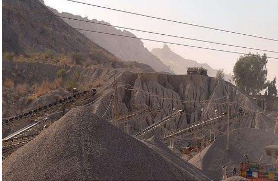
Figure 3.2: Margalla Hills Crush Plant
