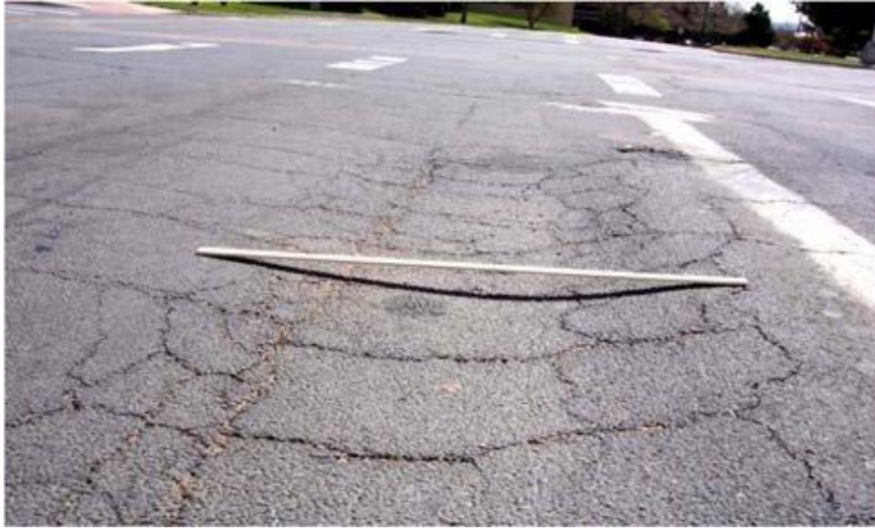
Figure 2.5 Rutting failure
