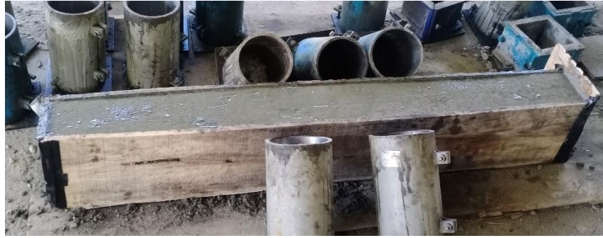
Figure 3.10 Casting of Concrete beam of span 1500 mm
