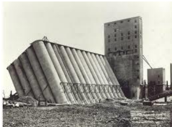
Figure 1.1 Failure of the Transcona Grain Elevator in October 1913 at North Transcona, Manitoba, Canada. (Obinna, 2021).
