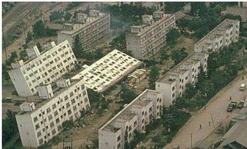
Figure 1.3 ground failure occurred due to the 1964 Niigata earthquake. (Wikipedia,2021)
