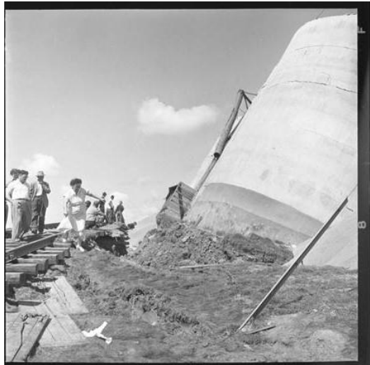
Figure 1.2 Failure of Fargo Grain Elevator 1956. (Olson,1955).
