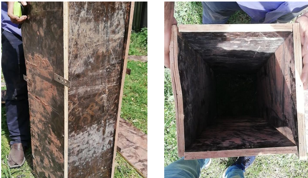
Figure 4 Mold used for Retrofitting (Phase-2 of Casting)
