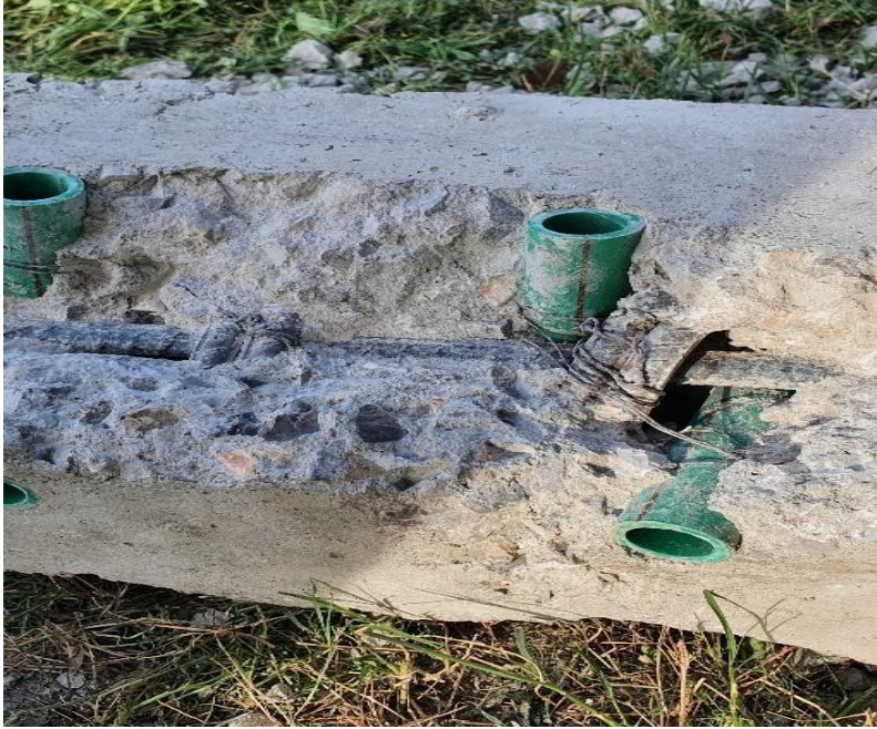
Figure 5 Prepared Surface (Removed Cover)
