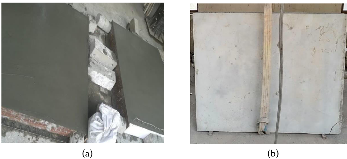
Figure 3.2.3: (a) and (b): Casting of 5' x 4' Slab Panel
