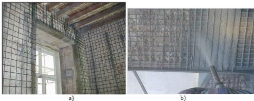
Fig. 10 a) Masonry wall from the inside with steel mesh, b) spraying of the cement grout into the wall [fotos by Appleton, 2011]
