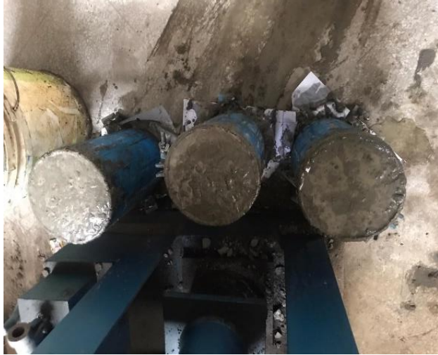
Figure 9: Casting of Cylinders
