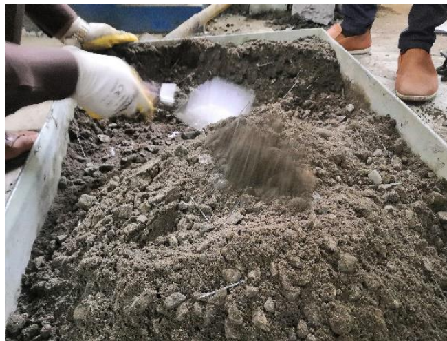
Figure 7: Mixing of Concrete
