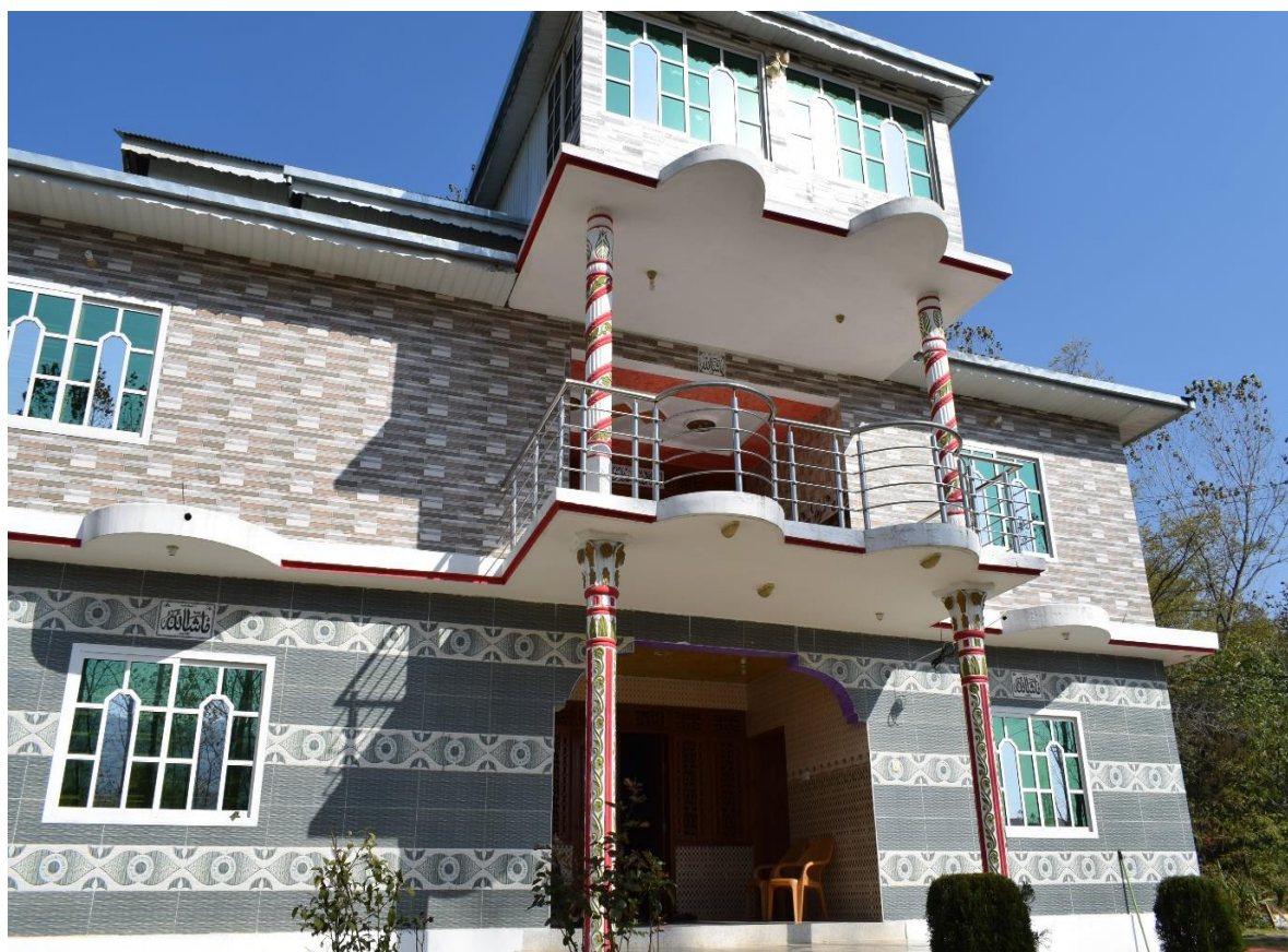
Figure 4.10 A multi-story house having hollow Ornamental columns as major load carrying members.
