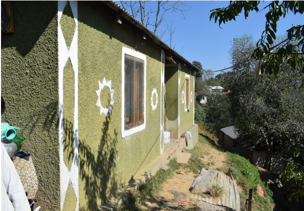
Figure 4.15 A house constructed on sloppy site
