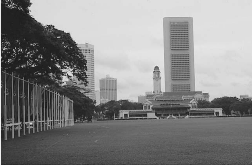
Figure 16.2 Singapore, a city state which, in spite of a dense population and a challenging humid tropical environment, has made impressive progress with urban environmental management. In a number of fields the city is among world leaders, notably in efforts to control car traffic and provide adequate public transport. The approach adopted has been quite 'top-down'.
