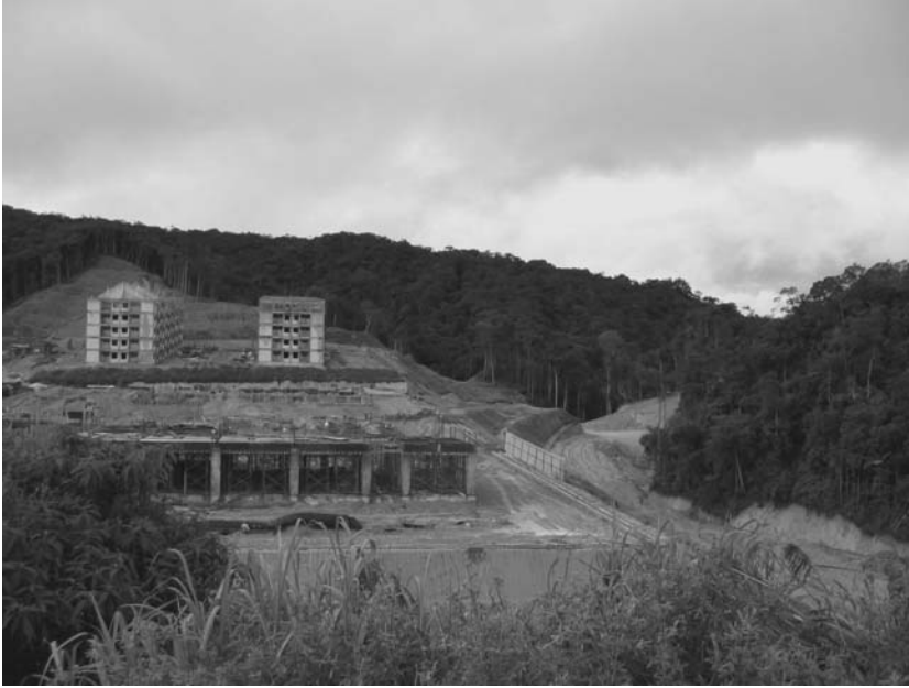
Figure 14.1 The development of apartments and hotels in the Cameron Highlands (Malaysia). Building on steep slopes threatens the valley with landslides and if great care is not taken silt and sewage will pollute streams. Along with unsustainable farming, this building destroys montane rainforest and occupants add to traffic and other pollution. Ideally this sort of development should be sited on already degraded land near the valley floor where it would do less harm to the biota and intrude less on the scenery.
