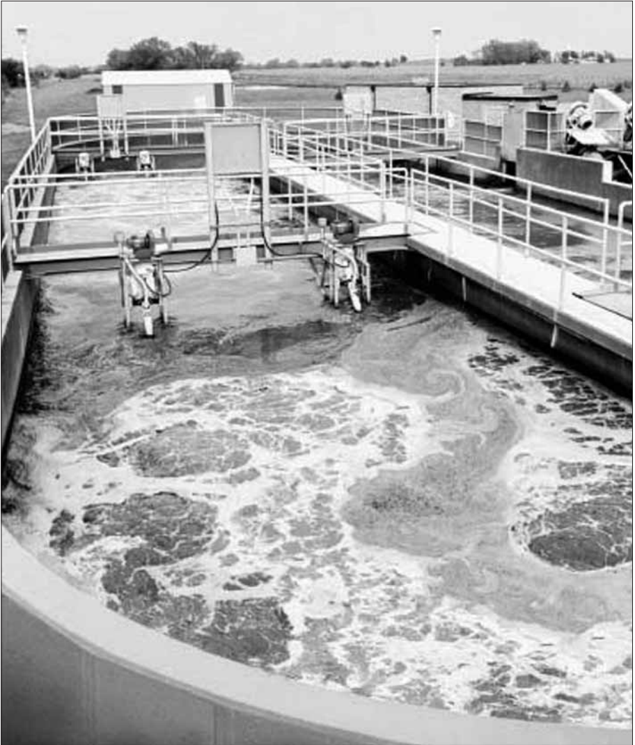
Figure 20.3 Typical Oxidation Ditch Installation
