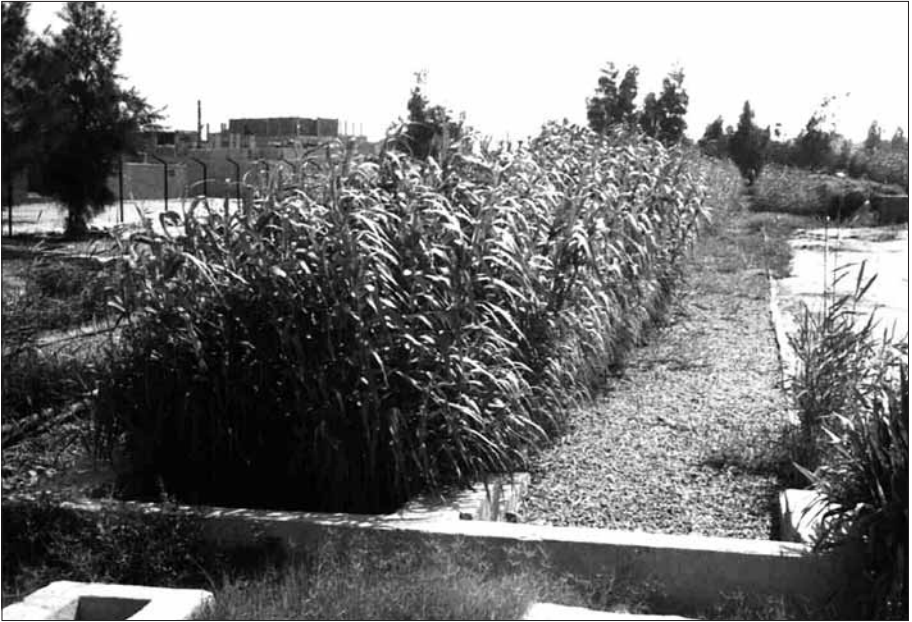
Figure 17.1 A 100-m Long Subsurface-flow Constructed Wetland in Egypt
