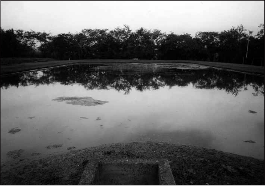
Figure 10.1 Anaerobic Pond, with Partial Scum Coverage, at Ginebra, Valle del Cauca, Southwest Colombia
