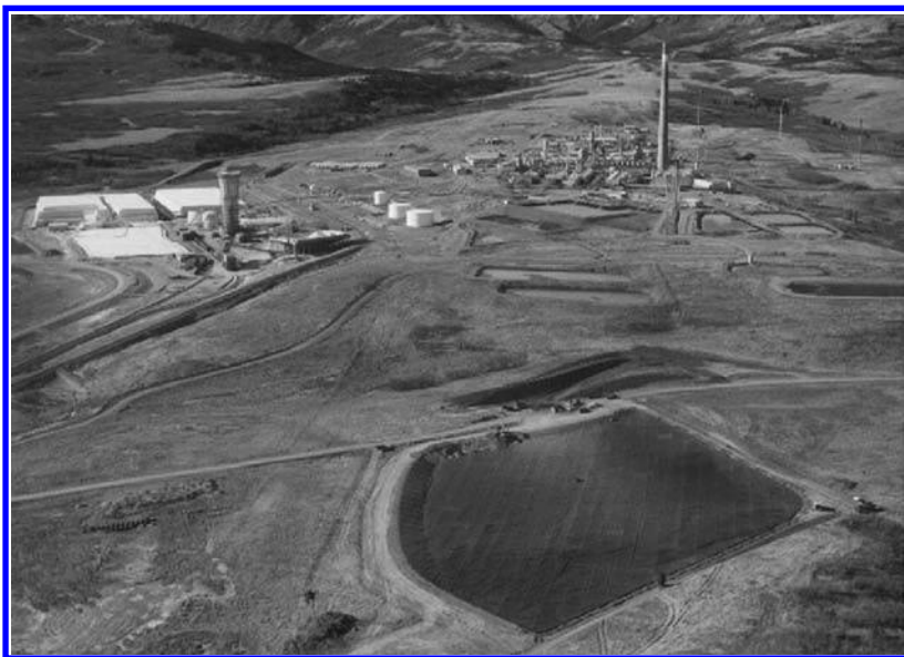
FIGURE 7.2 A newly constructed secure industrial waste landfill at a gas-processing plant. The landfill is lined and capped to prevent infiltration and generation of leachate. The landfill contains a variety of wastes generated by the facility over several decades, including contaminated soil generated during a major remediation effort at the site.
