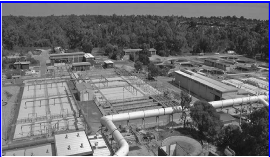
FIGURE 4.13 In some parts of the world, raw sewage continues to be discharged to natural watercourses. Wastewater treatment plants worldwide provide an essential service, without which the natural environment and human health would suffer significantly. However, as we seek to improve levels of treatment by upgrading existing facilities or setting even more stringent water quality standards to achieve even greater gains in environmental protection, costs rise. (Photo courtesy of WorleyParsons.)
