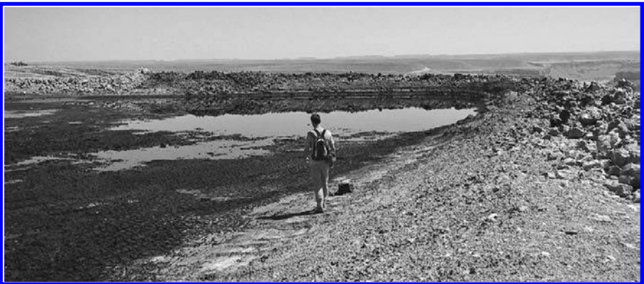
FIGURE 4.1 Oil exploration wastes in an unlined open pit. Oil and produced water may seep into shallow groundwater, causing contamination.
