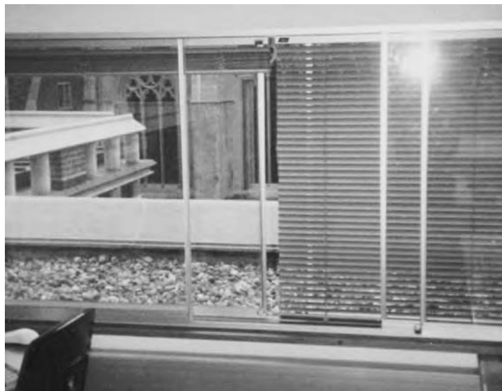
4.5 Venetian blinds in the cavity of a double window.
