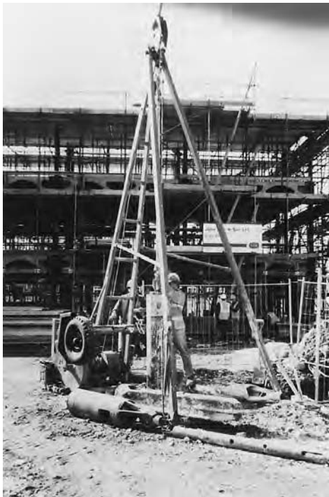
14.7 Borehole drilling rig.
