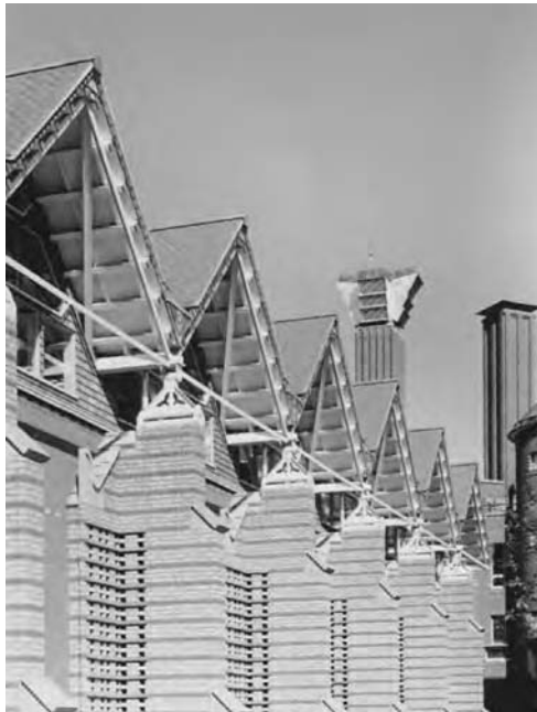
12.7 Mechanical laboratory showing buttress side wall vents with classroom exhaust stack and boiler flue behind.
