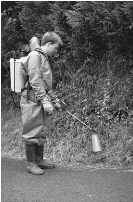
Fig. 3.12 (Continued.) (b) Spraying pavement to control weeds; (c) with shield around nozzle to protect spray from wind. (Continued.)
