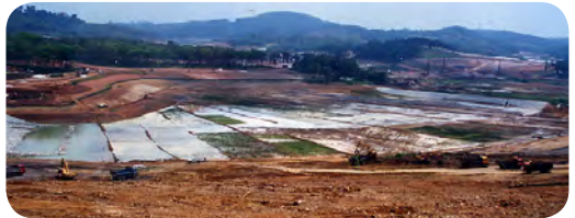
A complete constructed wetland cell
