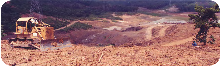
Clearance of existing vegetation to construct a wetland landform
