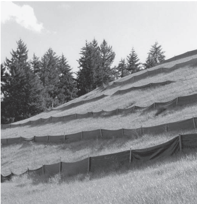
Silt fences and grass stabilization at a construction site
