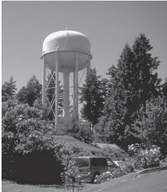
Water storage tower
