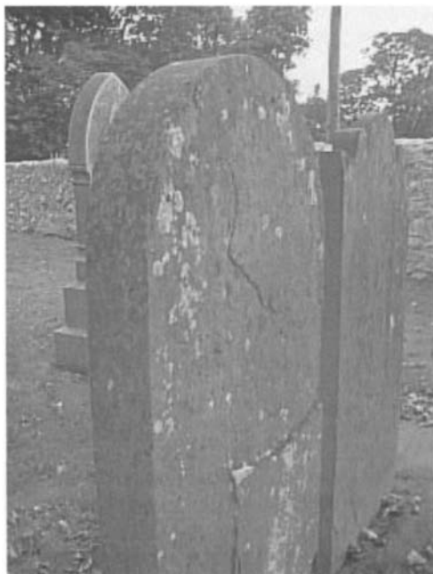
Figure 3.5 Decay of building stone owing to air pollution in northern Scotland (courtesy of the Scottish Environment Protection Agency (SEPA, 2000))
