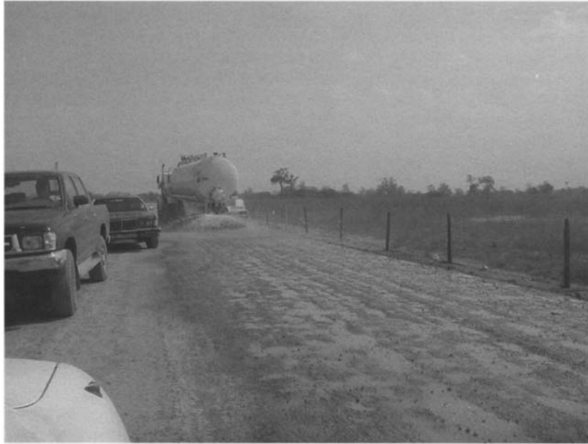
Figure 8.1 Fugitive dust emission control in eastern Venezuela (courtesy of Perez Companc SA)
