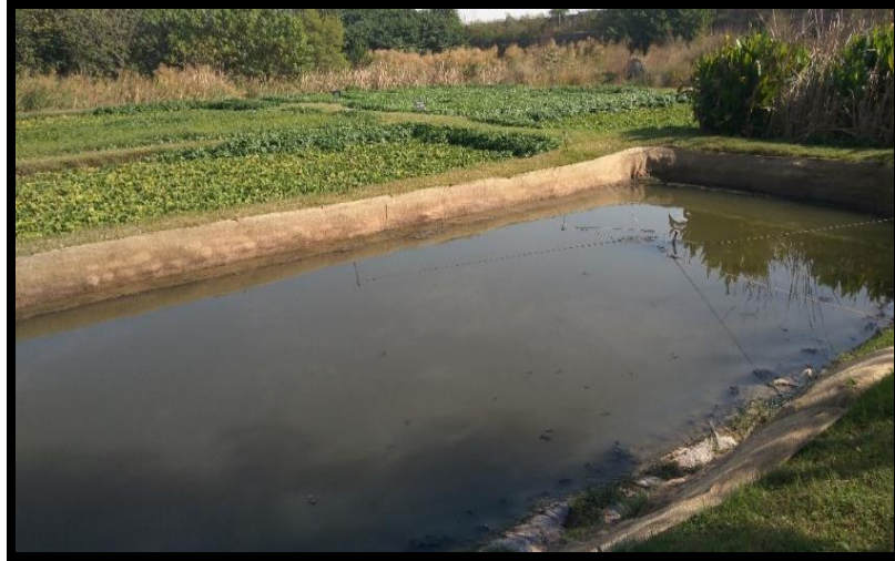
Figure 7: Integrated Constructed Wetland System (ICWs), NUST Islamabad
