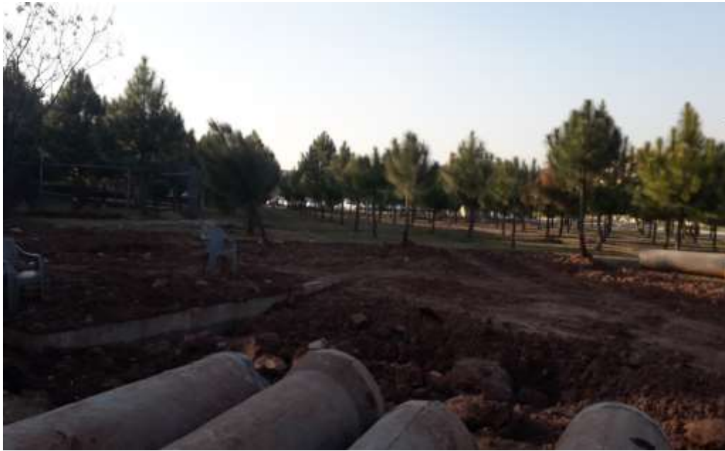
Figure 3-4 Construction process of RCC Storage Tank
