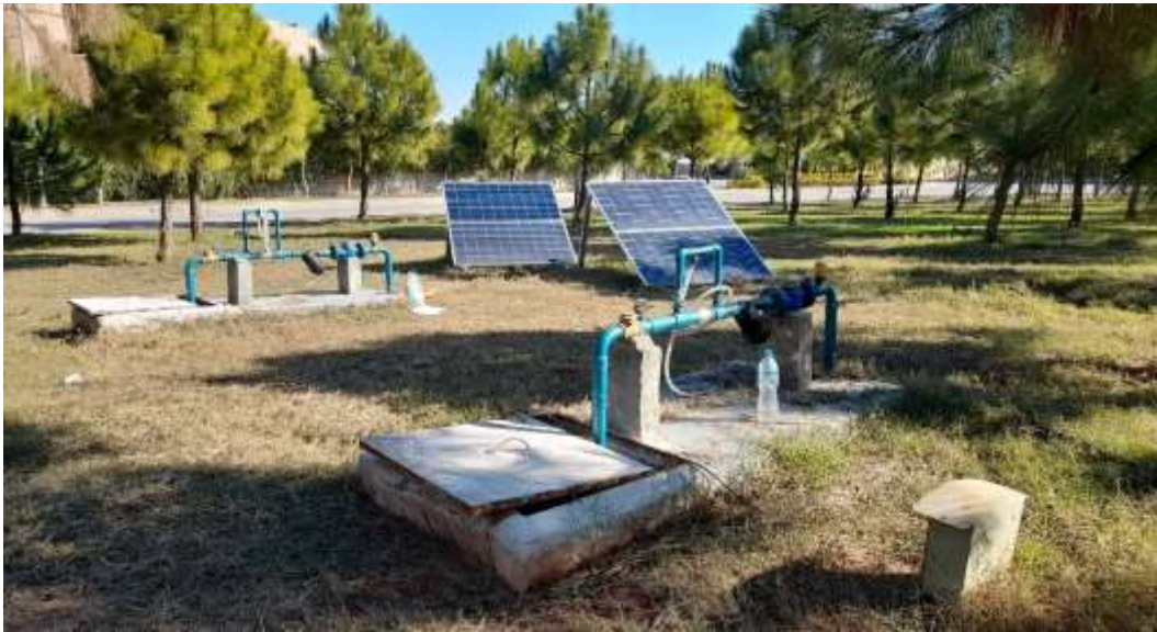
Figure 1-1 Rainwater harvesting pressurized irrigation (RWHPI) model installed at NUST Business School (NBS)
