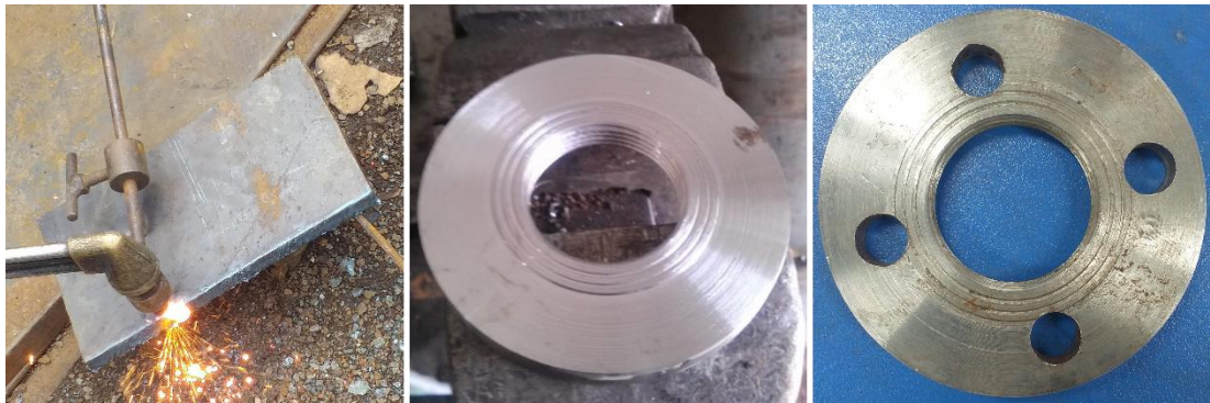
Figure 3.4 Fabrication of Flange
