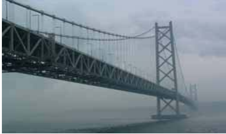
Fig. 2.1. Akashi-kaikyo bridge,Japan, using SCC
