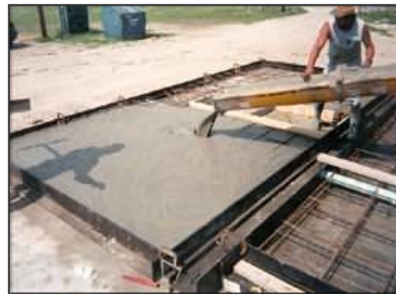
Fig. 1.2. Casting of Foam concrete in panels (Litebuilt 2005)
