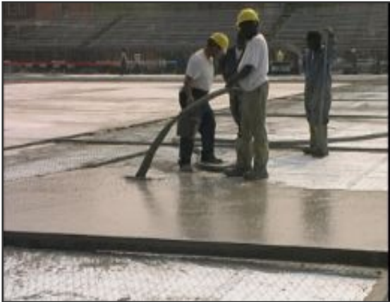
Fig. 1.3. Casting of Foam concrete for roof insulation
