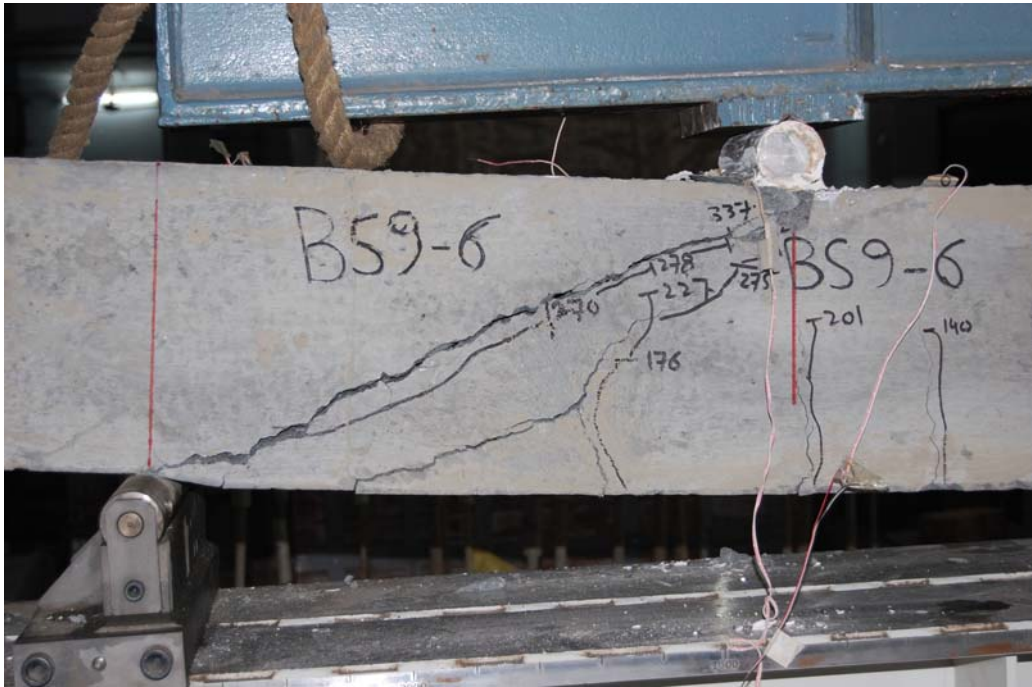
Fig 4.17 (b) Cracking pattern BS 9-6
