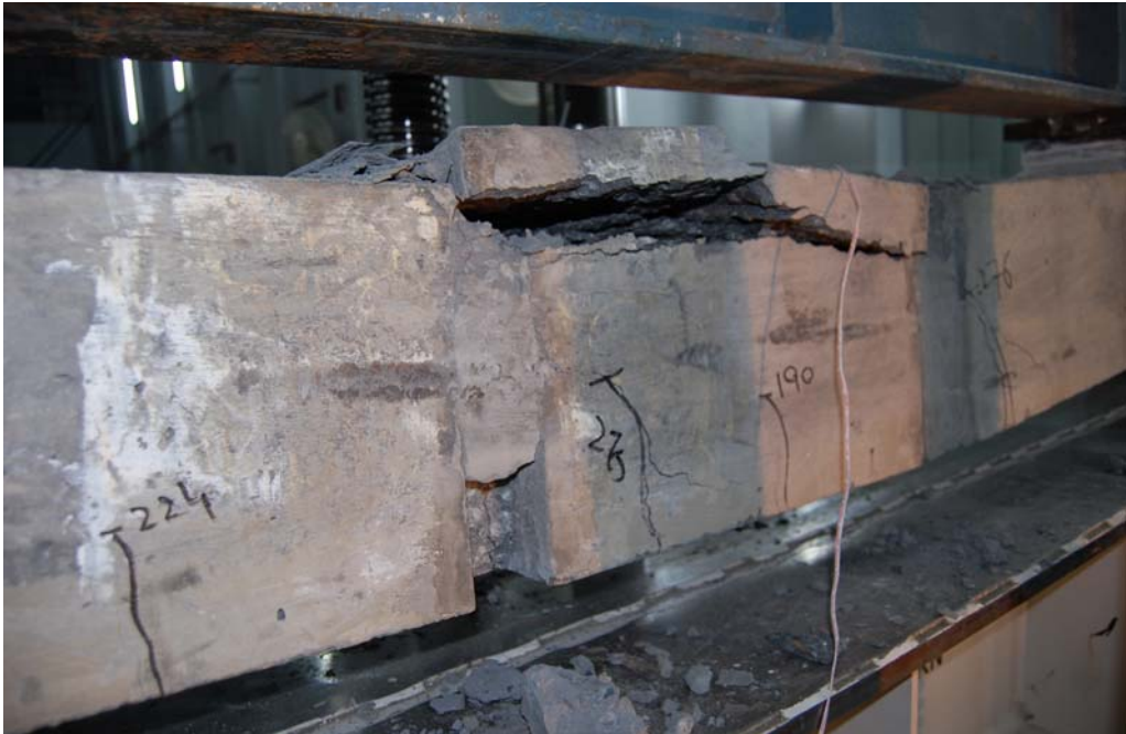
Fig 4.16 (a) Cracking pattern BS 9-5
