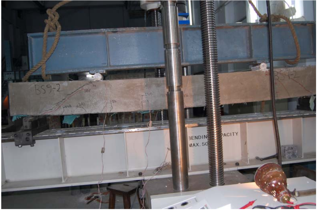
Fig 4.13 (b) Cracking pattern BS 9-2
