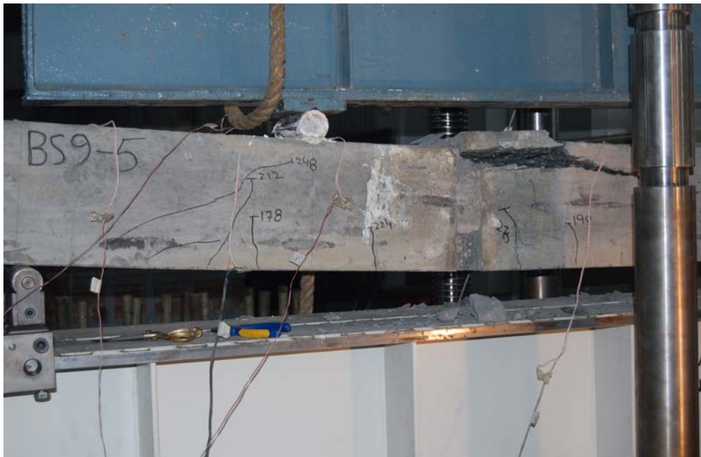
Fig 4.16 (b) Cracking pattern BS 9-5
