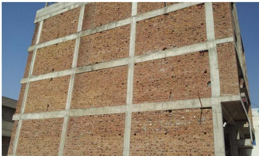
Figure 2.1: Brick masonry infill with concrete frame.
