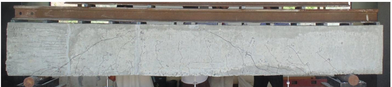
Figure 4-6: Cracked Pattern of N-1
