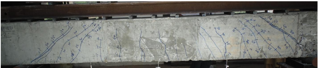
Figure 4-21: Cracked Pattern of MZ-II
