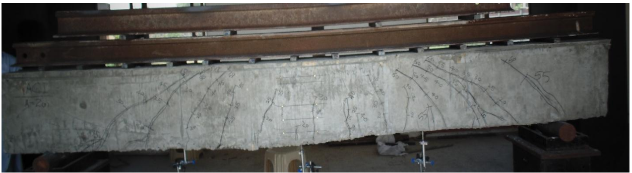
Figure 4-12: Cracked Pattern of ACI-II
