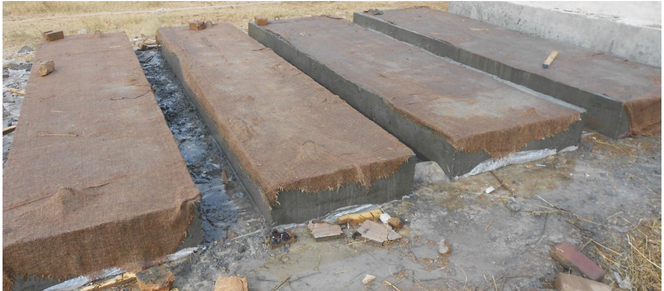
Fig3.3 Curing of Beams
