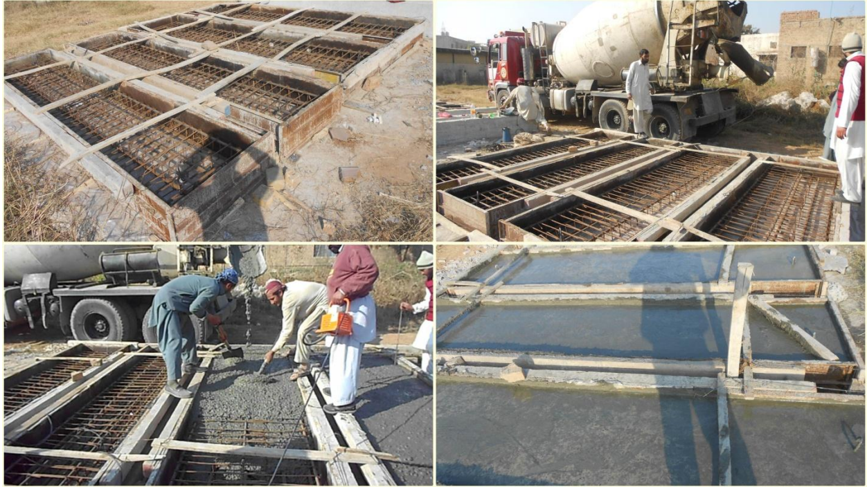
Fig 3.1-Casting of Beams at NICE, NUST, Islamabad.
